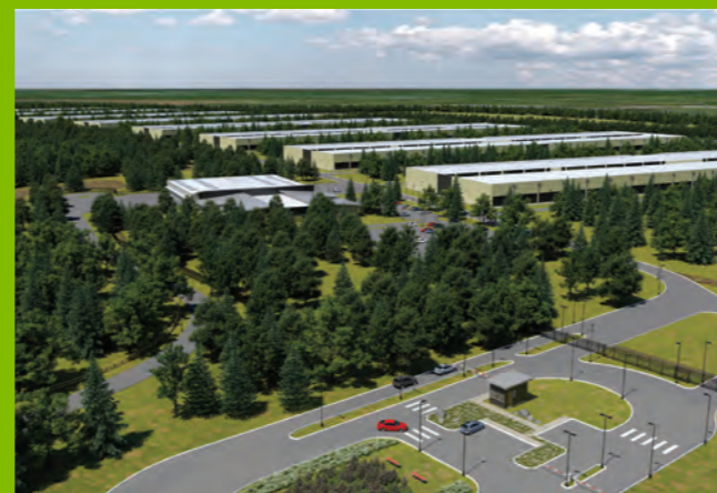
Recent announcement by APPLE to locate its Data Centre in the West of Ireland
